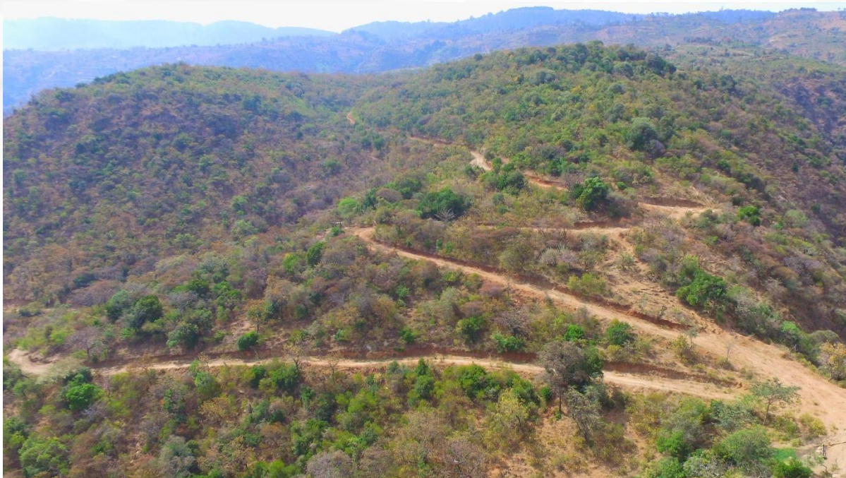
Figure 23. Improved road access
