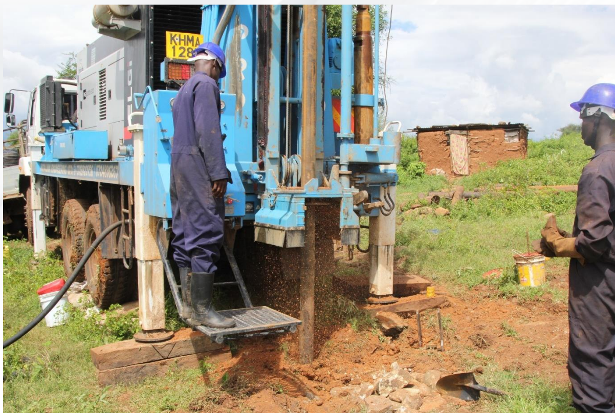
Figure 24. Drilling of Boreholes
