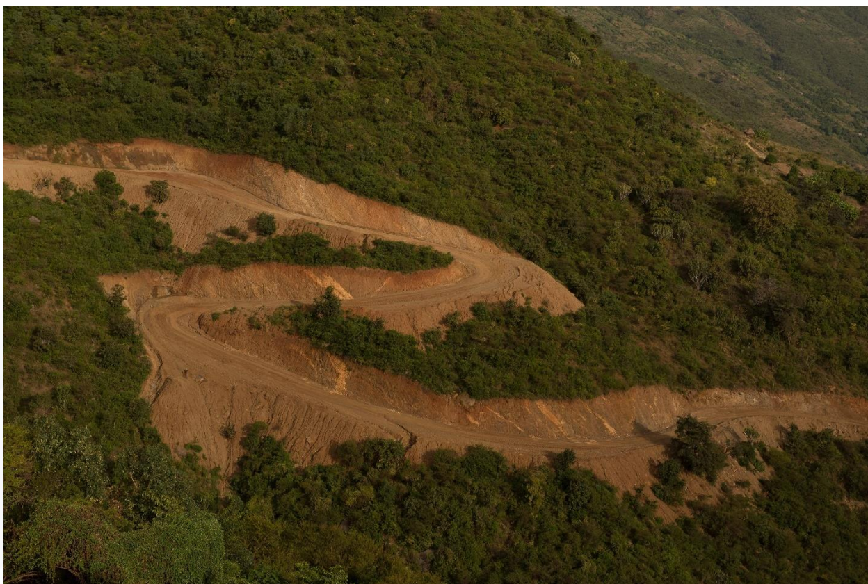
Figure 8. New road across the escarpment
