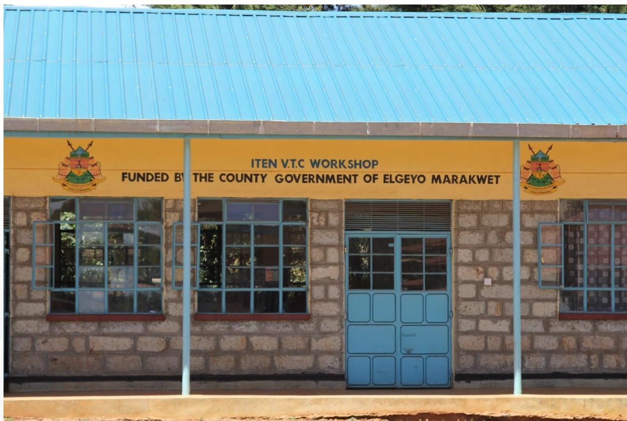
Figure 9. Upgrading of Iten VTC
