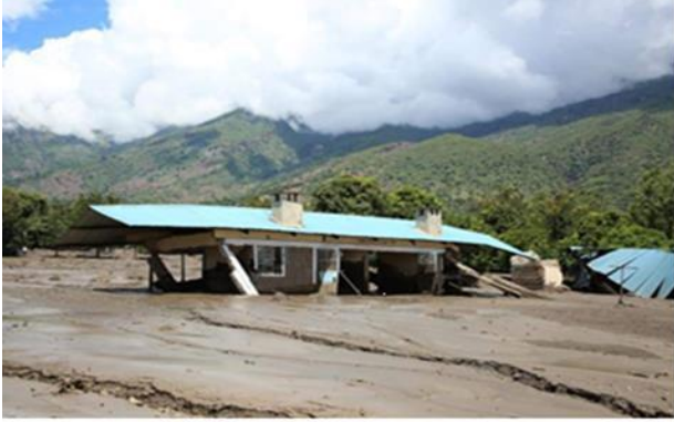
Floods at liter girls high school, Endo Ward 2020
