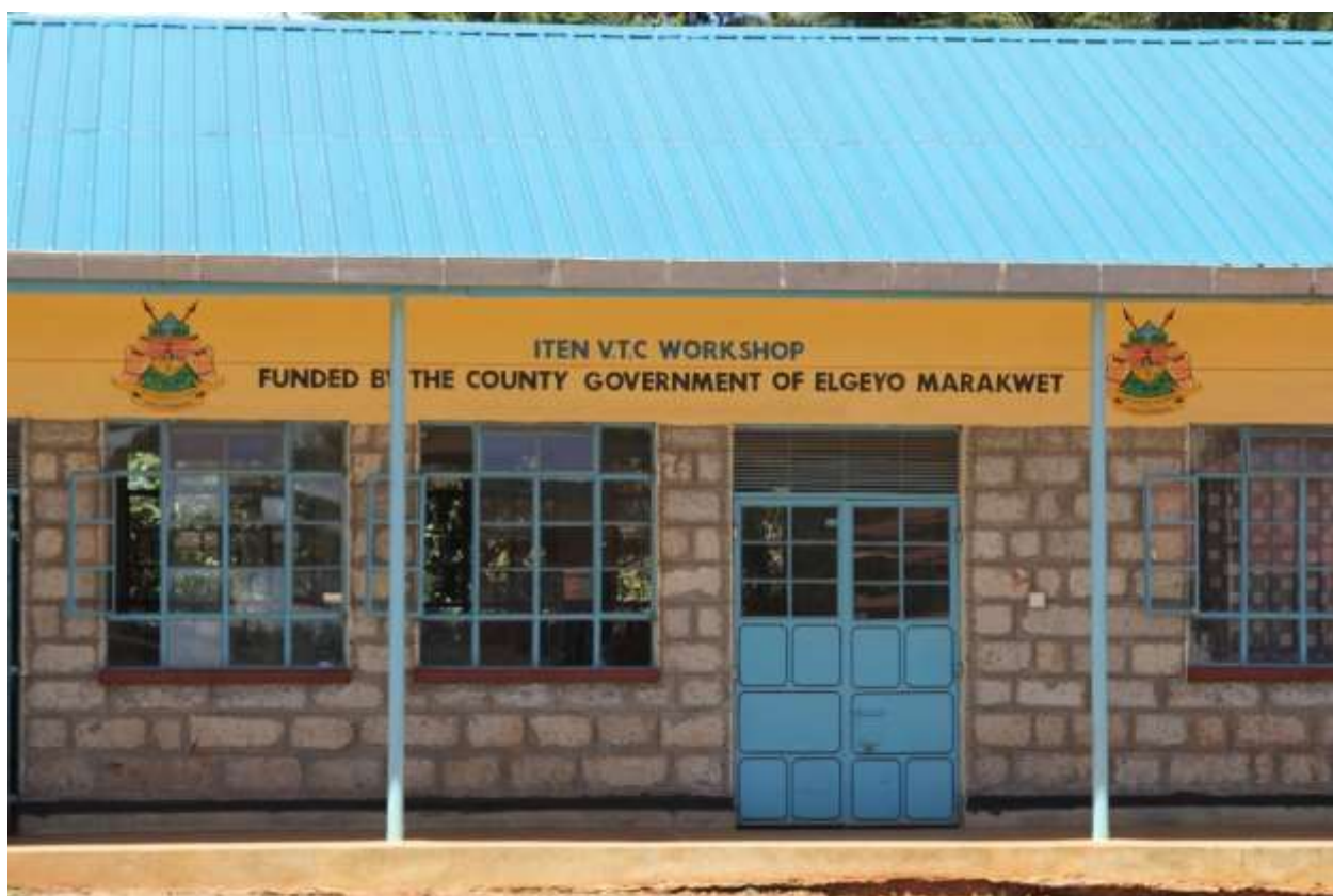
Figure 9. Upgrading of Iten VTC
