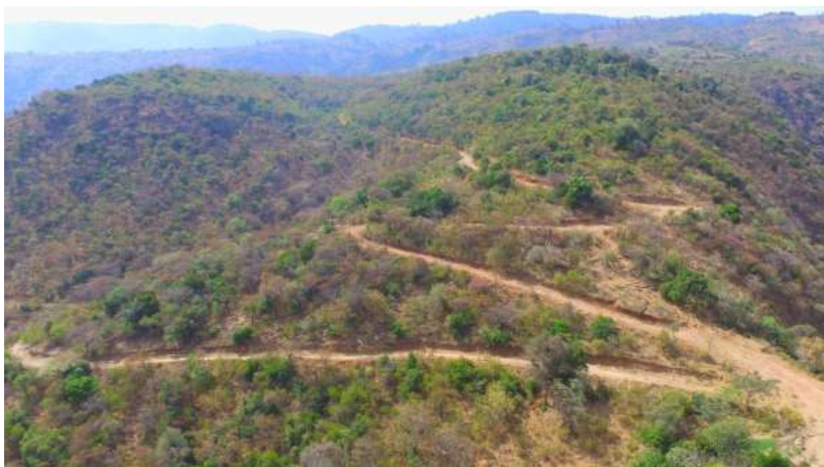
Figure 23. Improved road access
