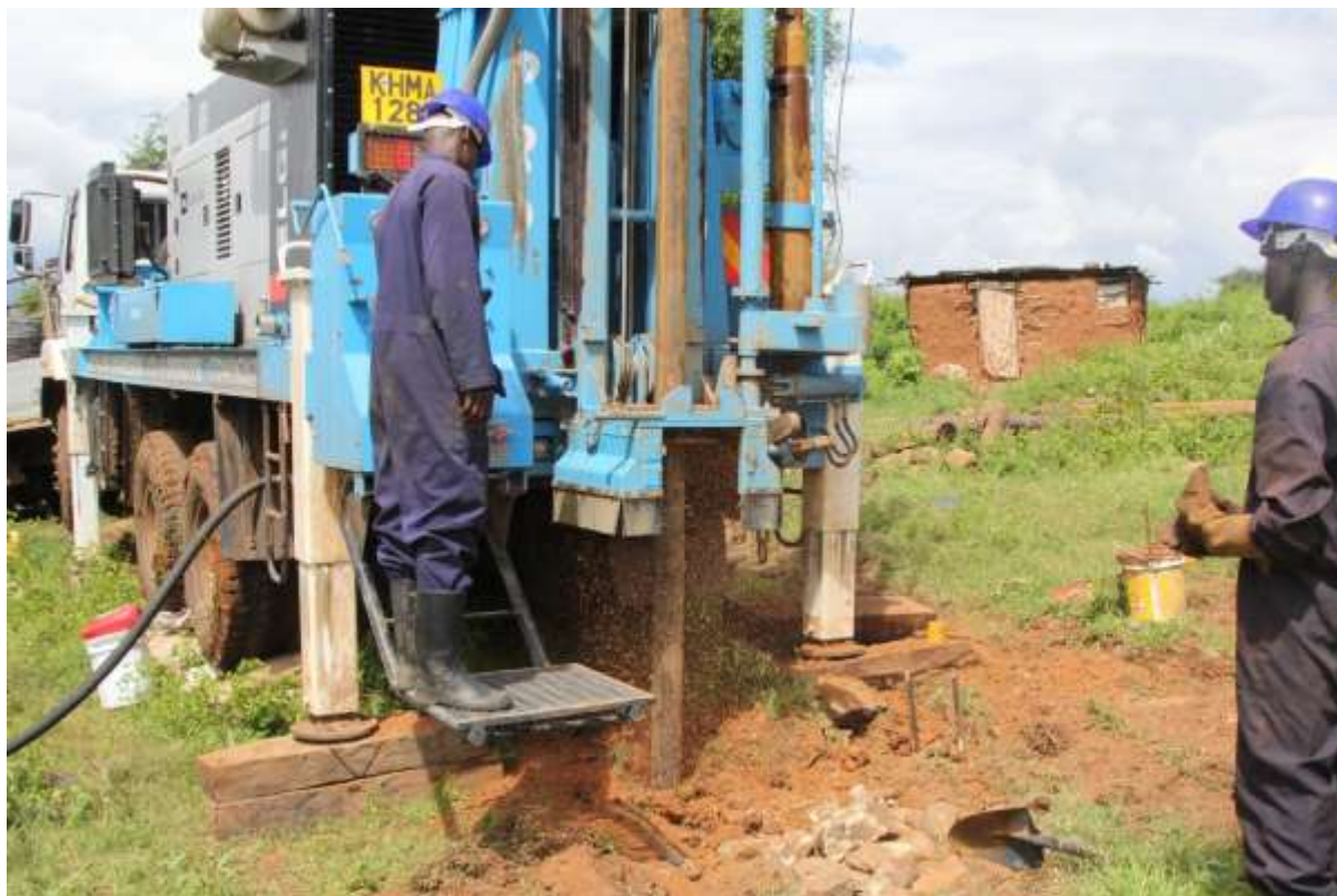
Figure 24. Drilling of Boreholes
