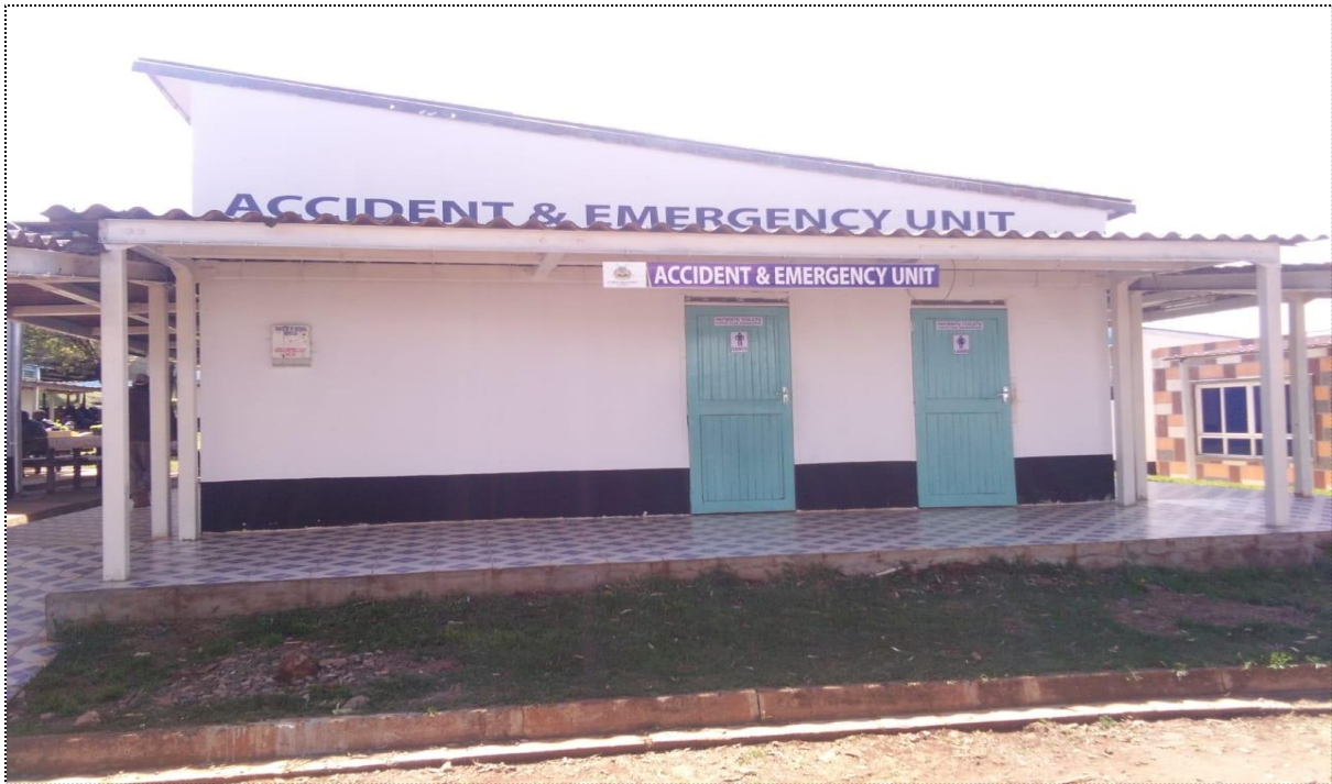
Iten County Referral Hospital Accident and Emergency Unit, construction complete and operational.
