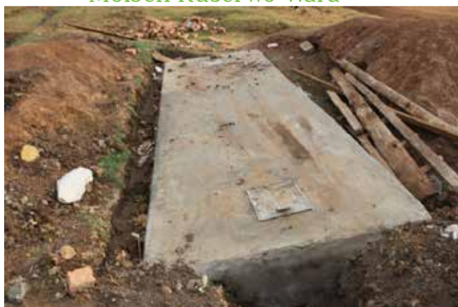
Cheptongei milk cooler project Septic Tank PHOTO | GPSU
